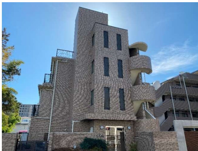
Tachikawa headquarters office building (2 nd floor)
